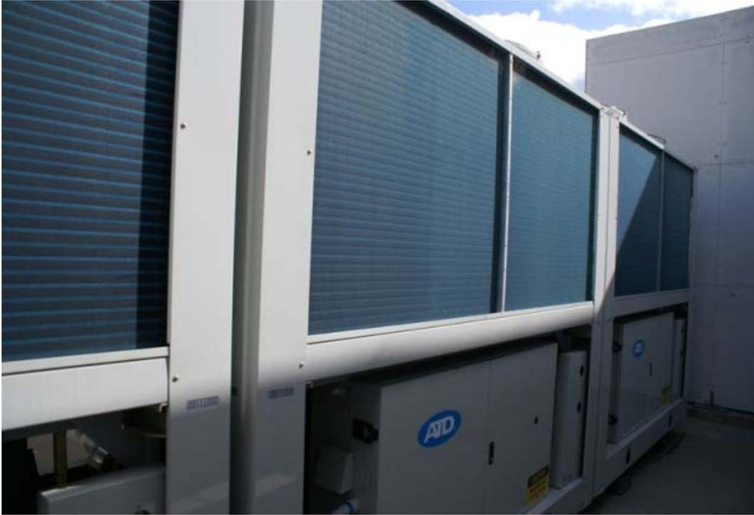
Three 750kw Air cooled water chiller package. Model: LAAWCPB750
